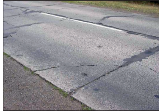
Fig. 2. Transverse cracks in the slabs and corners [1]
