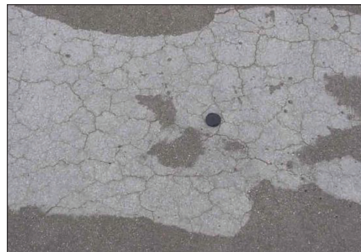
Fig. 4. Surface defects, alkaline cracks [1]
