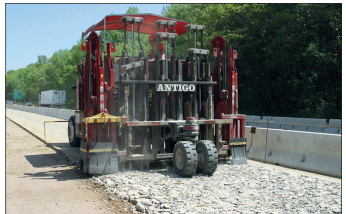
Fig. 17. Multi-head breaker 0 [13]
