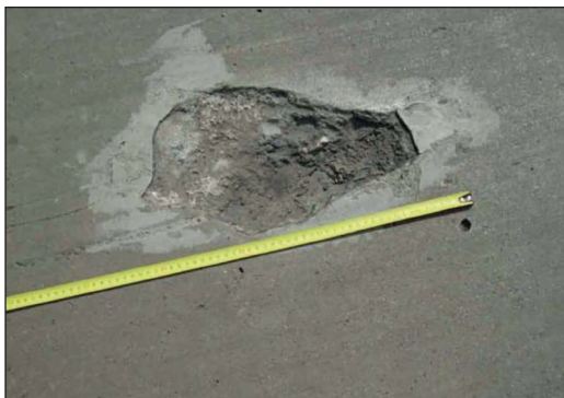
Fig. 4. Surface defects, alkaline cracks [1]
