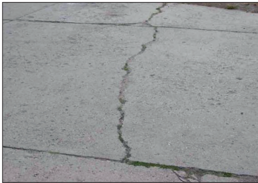
Fig. 3. Longitudinal and transverse cracks (fractured slab) and near-edge cracks [1]
