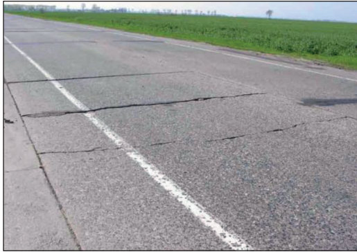
Fig. 2. Transverse cracks in the slabs and corners [1]
