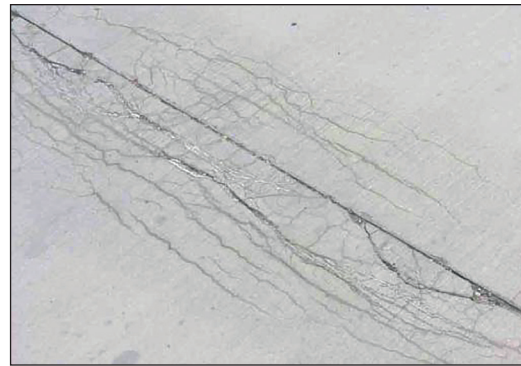
Fig. 3. Longitudinal and transverse cracks (fractured slab) and near-edge cracks [1]
