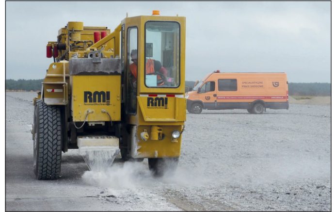
Fig. 18. Resonant pavement breaker; photo by the author
