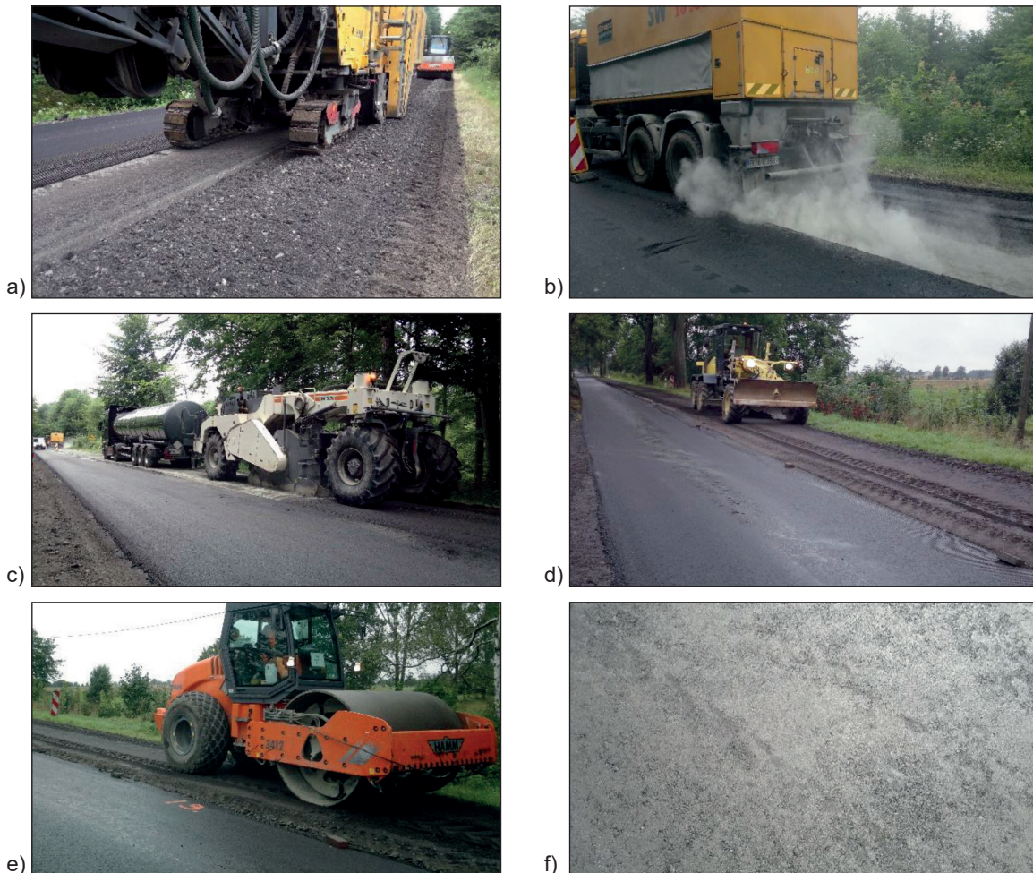
Fig. 2. Preparation of the field sections located on the Voivodship Road No. DW 172
