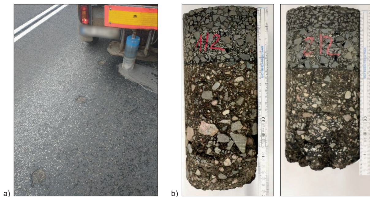
Fig. 5. Cores obtained from the field sections after 10 years of exploitation: a) exemplary location of the coring, b) examples of the field cores drilled 10 years after compaction
