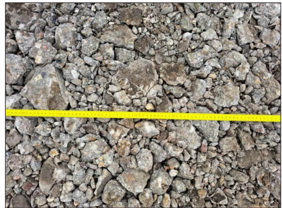
Fig. 4. Measurements of the geometric dimensions of the fractured concrete rubble [9]
