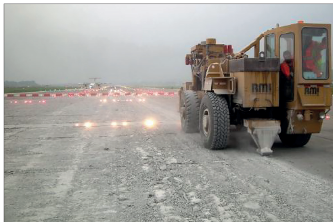
Fig. 3. Machine for ultrasonic rubblizing RMI [4]
