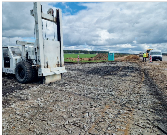
Fig. 2. The self-propelled concrete guillotine GPB [9]
