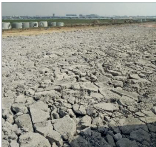
Fig. 6. View of the stress-relieved cement concrete layer on one of the test sections [9]
