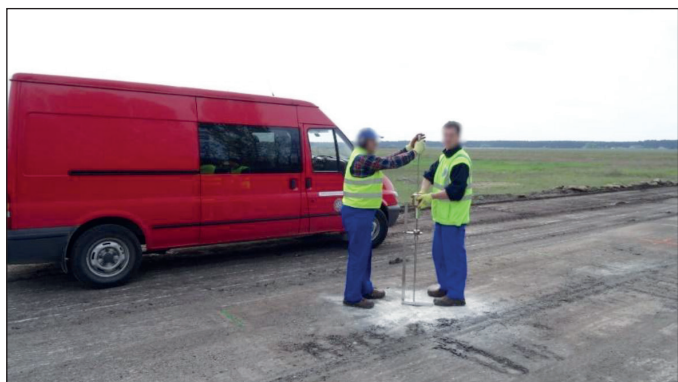
Fig. 7. Subgrade bearing capacity testing with the DCP probe on one of the test sections [9]
