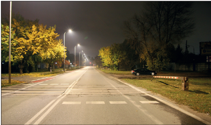
Fig. 1. Roadway lighting with designated bike lanes
