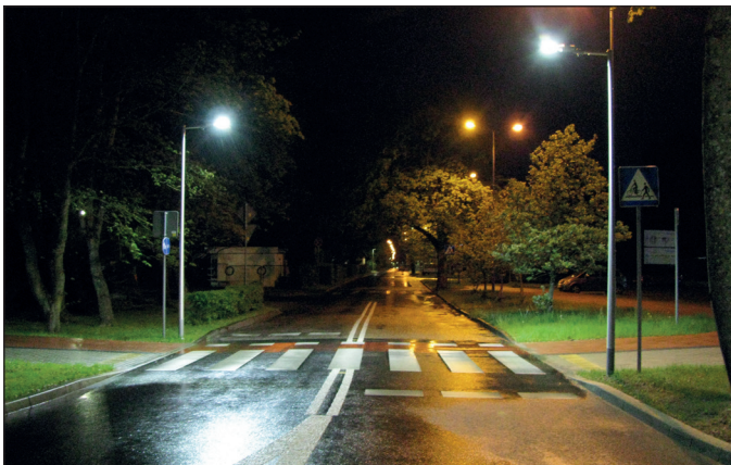
Fig. 5. An example of lighting a bicycle crossing including a pedestrian crossing using a dedicated solution (PC class)
