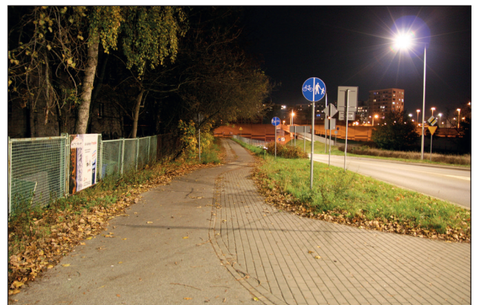
Fig. 4. Examples of lighting pedestrian-bicycle road with the same lighting fixtures
