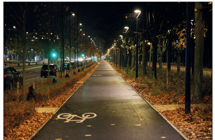
Fig. 3. Examples of lighting bicycle road with separate luminaires
