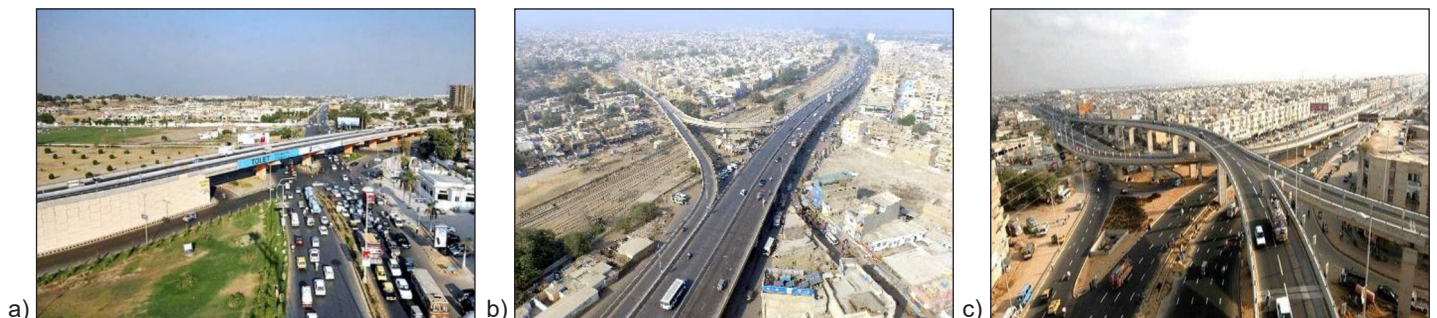
Fig. 2. Existing identified case-study bridge: a) bridge I, b) bridge II, c) bridge III
