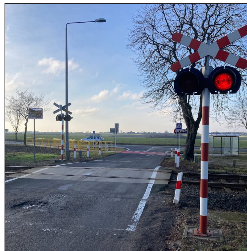
Fig. 2. Railway level crossing with an automatic user-side warning (category C) with pavement made of large-size reinforced concrete crossing slabs
