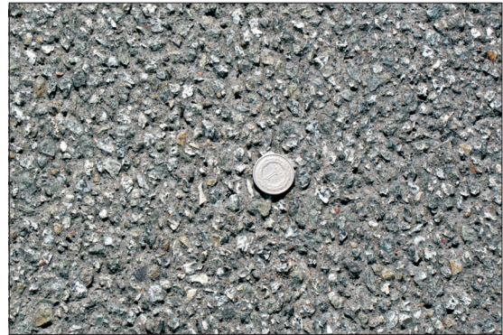
Fig. 3. Exposed aggregate concrete produced using gabbro aggregate on the Section B
