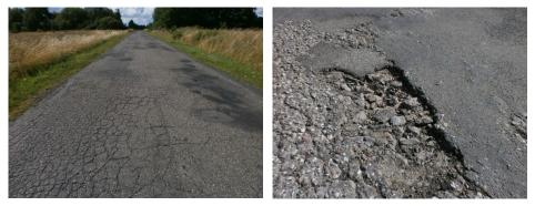
Fig. 1. A bituminous pavement affected by cracking and ravelling
